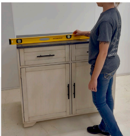
Check front-to-back and side-to-side level of case.
