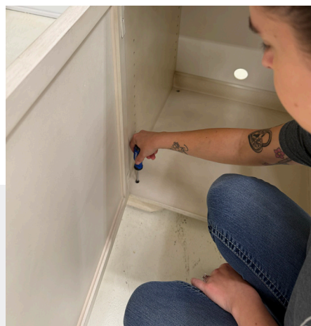
Use flathead screwdriver to adjust leveling glides from inside case.
